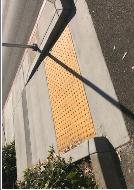
Curb Ramp Construction
